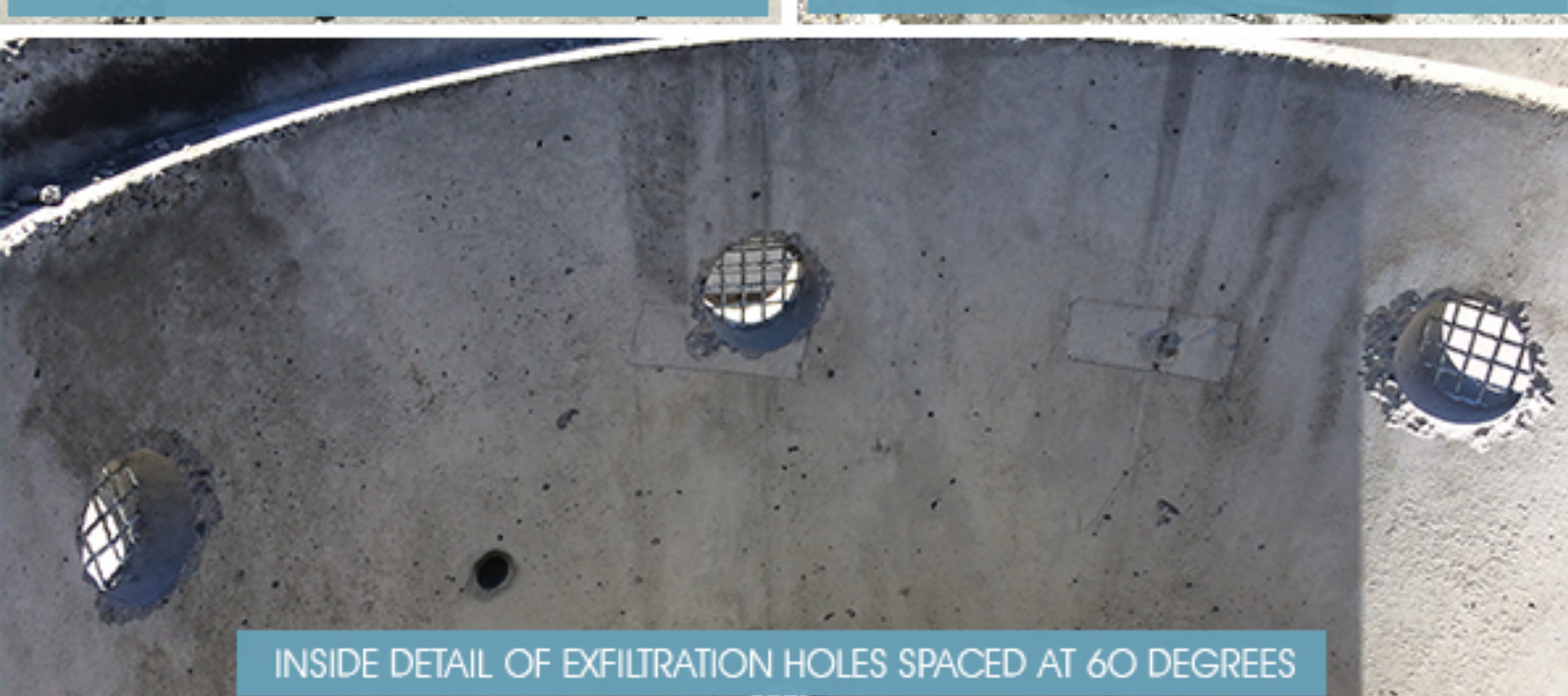
CAST EXFILTRATION HOLE DETAIL
