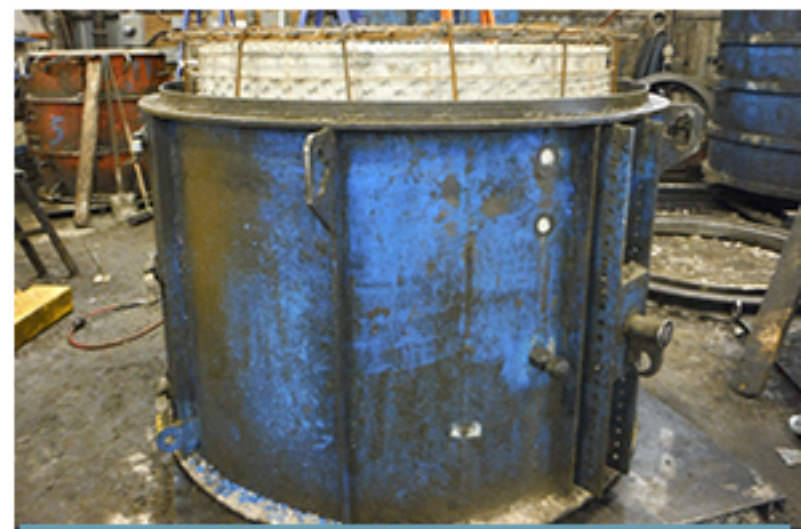
SETUP PRIOR TO POURING
