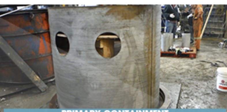
PRIMARY CONTAINMENT 5mm 316 STAINLESS STEEL
