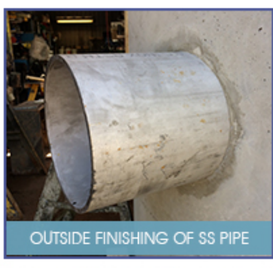
SS PIPE PENETRATION WELDING
